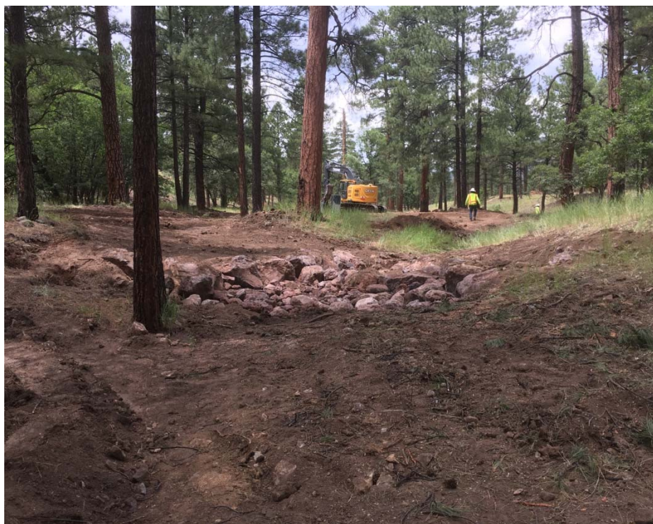
Cross-vane weir grade control upstream of Paradise Road
